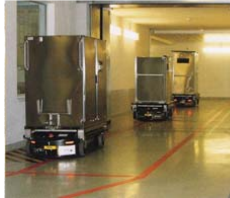
Automatic guided transport system. Every day about 800 rides in the new complex
